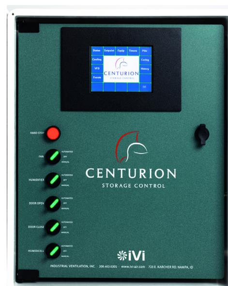
*Industrial Ventilation placed the Reach 5.7" Hitachi Enclosed Unit front and center on the main control panel of their Centurion product line.*
